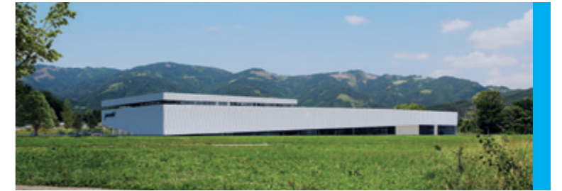
The new High-Tech and state of the art Aerospace plant in Kapfenberg.
